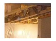
The lighting in the basement areas is incandescent lighting, operated by pull strings and wall switches. The basement lights were operational at the time of the inspection. The receptacles in the basement are grounded receptacles. The receptacles were tested and found to be properly wired.
